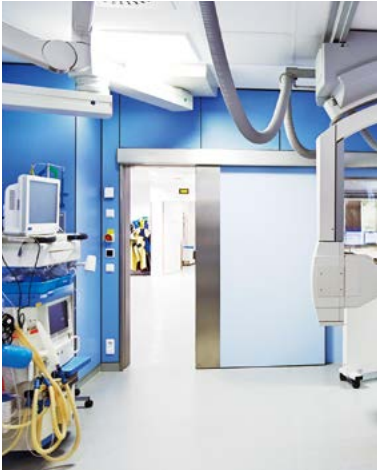
Doors for functional rooms
